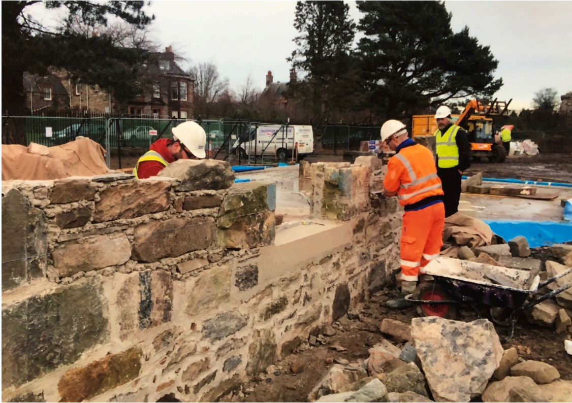
Fig 26: Construction on the Cottage re-used as much original material as possible (Image courtesy Botanic Cottage).
