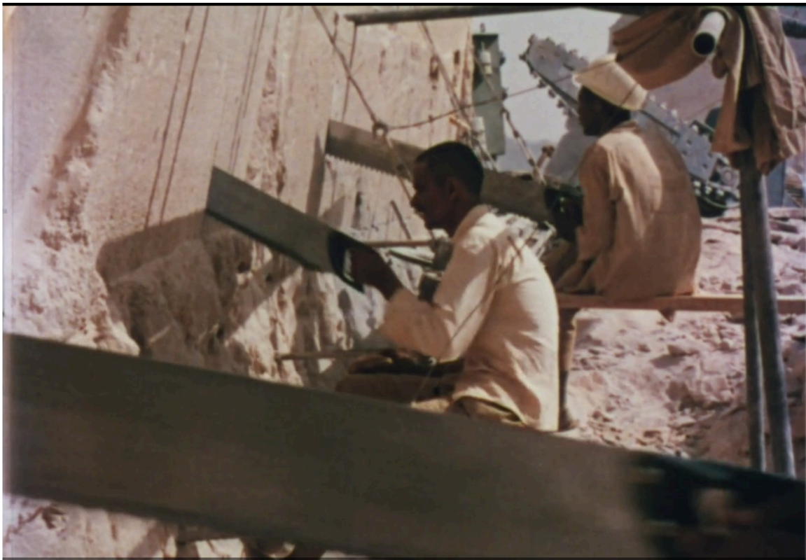
Fig 7: Workers saw the Abu Simbel into blocks to be moved. (From UNESCO 1968)
