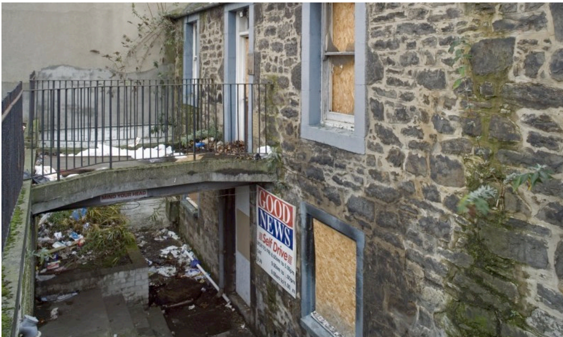
Fig 21: Exterior view of the front of the Cottage showing the rise in street level. The original first floor has now become the ground floor (From GUARD 2009, accessed via Canmore: 037323).
