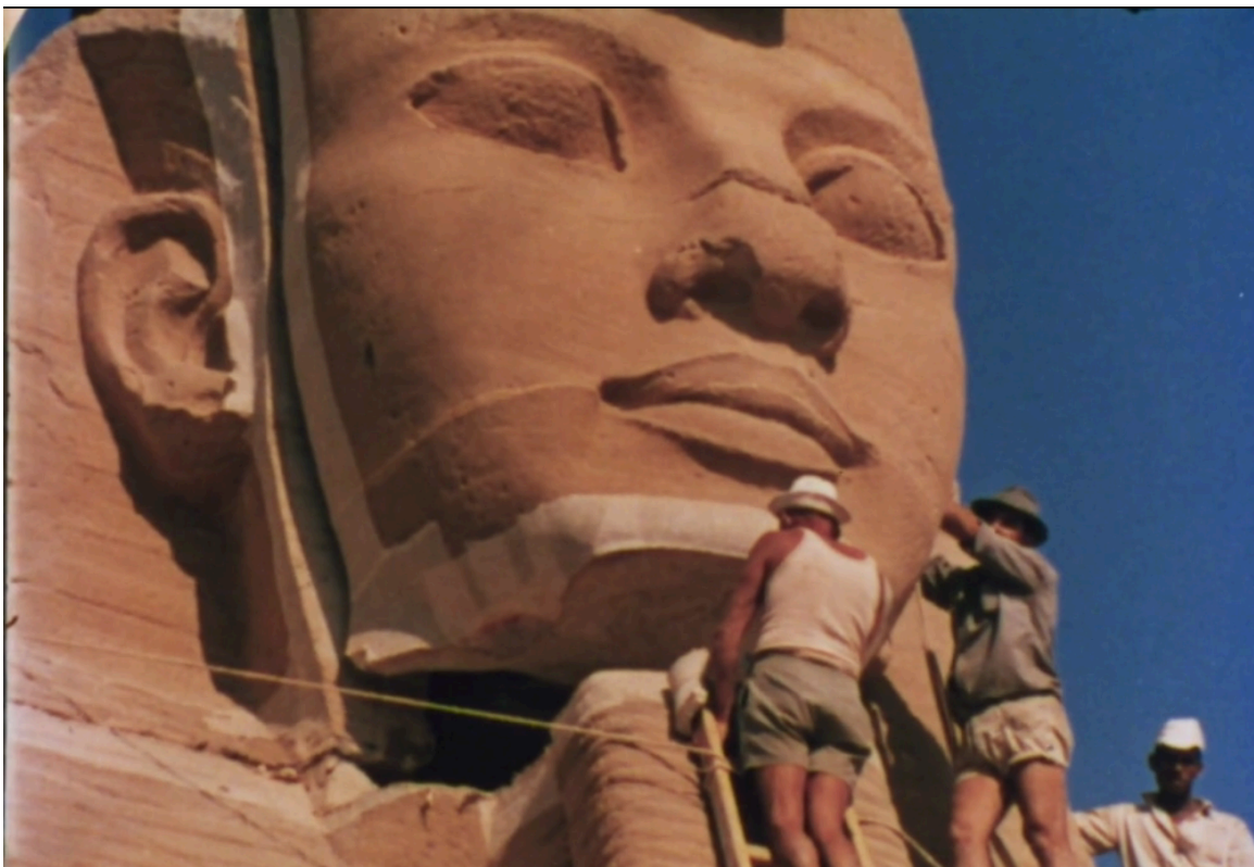
Fig 9: Workers remove the cut face of a statue of Ramses II (From UNESCO 1968).
